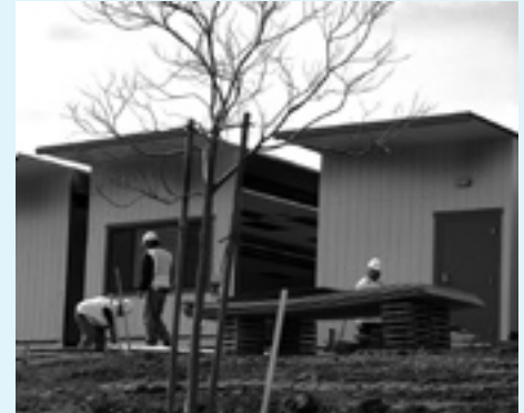
New portable buildings will house classes and labs during renovation
